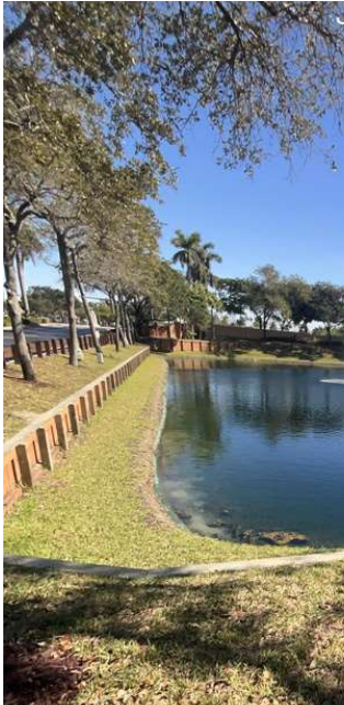
Lakes 4 & 5 - Showing the completed shoreline restoration from Phase 1 and the current wooden retaining walls to be replaced by the Prolock Omega Retaining wall
