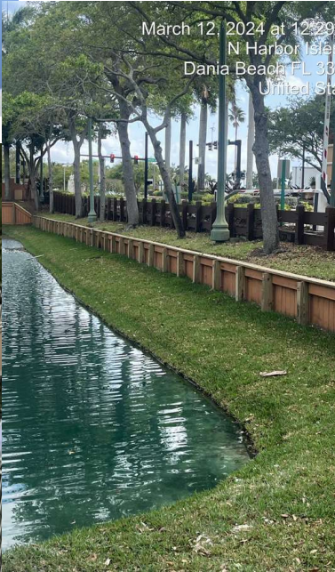
Lakes 4 & 5 - Showing the completed shoreline restoration from Phase 1 and the current wooden retaining walls to be replaced by the Prolock Omega Retaining wall
